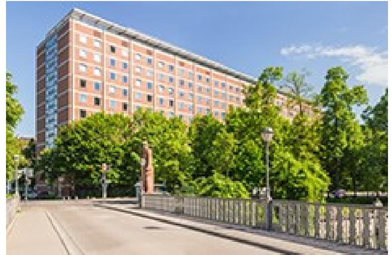
GPTO headquarters in Munich
