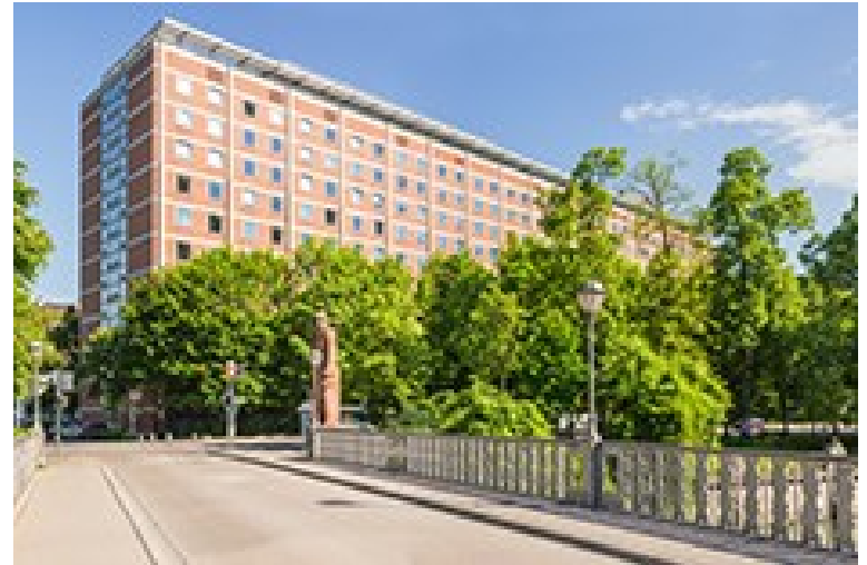
GPTO headquarters in Munich
